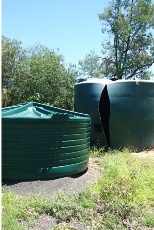
Terpersie tanks Large one split asunder and all water lost.
